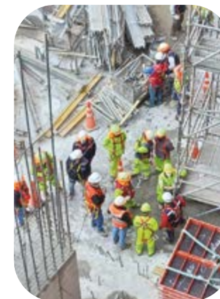
ONSITE INTERVENTION: "HOISTING WORKSHOP."
